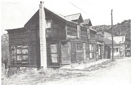
FIGURE 2-38. A cement block chimney intrusion on this building (Block 2, Lot 31).
